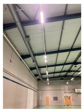
Yarls Wood detention centre sports hall required lighting upgrade IDWE asked ALD to propose a new scheme using LED we proposed our SP60 sports lighter which was ideal for the application as these were to be mounted on lighting trunking
