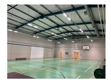
Within this scheme we used a total of 15 x 114w luminaires each luminaire having 60° optic and wire protection grill to prevent damage from Footballs & Basket Balls
